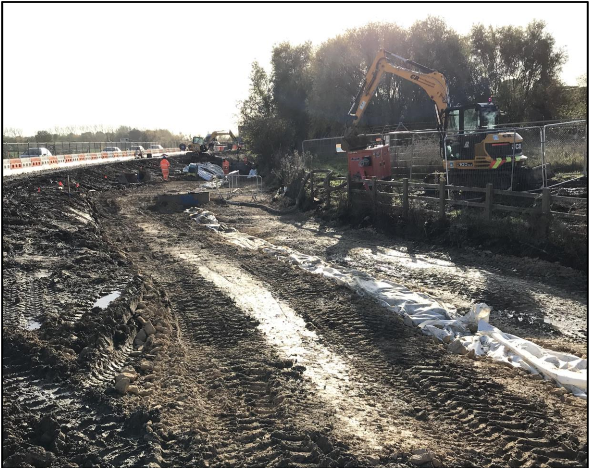
Springfield Road Roundabout South West Quadrant
