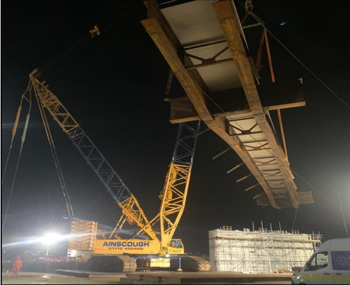
SWRR – 1 st Braced Beam Commences Lift
